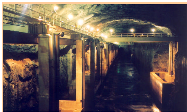
Figure 19. Tailrace surge chamber.
