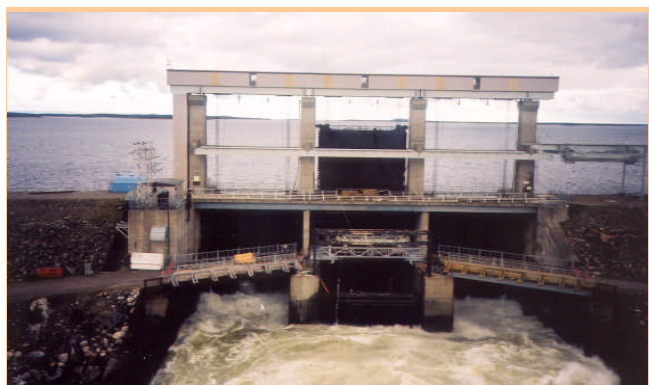
Figure 18. Lobstick flow control structure. Stoplogs in place for repairs to middle sluice.
