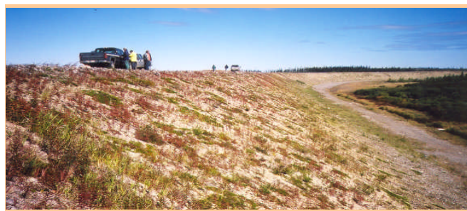
Figure 20. Typical dyke. Total crest length = 64.4km.
