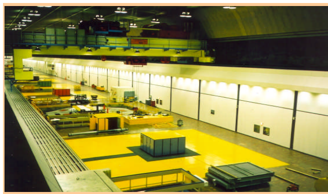
Figure 17. Underground powerhouse generator floor. 11 units, total capacity 5,428MW. Length = 296m. Height = 47m. Width = 25m.
