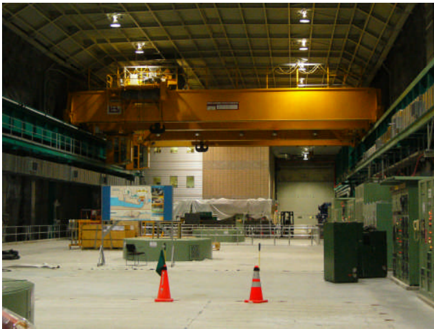
Figure 1. Generator floor, Peribonka powerhouse. 3 Francis units, of 128MW at 67.6m rated head.
