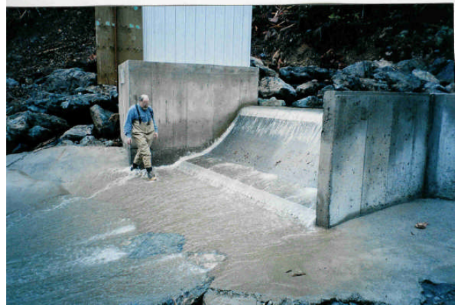
Figure 3. 4.5MW Marion creek, BC. 1.1m 3 /s Coanda intake, head = 495m. (Source - Pentti Sjomani, P.Eng.)
