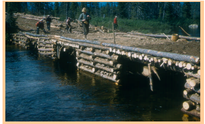
Figure 9. Typical timber crib bridge on access road.
