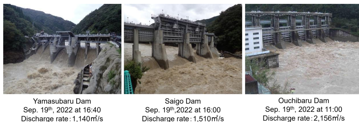
Figure 4-24 Picture of the 3-Dams Coordinated Sediment Flushing Operation
