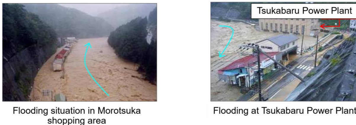
Figure 4-9 Status of Flooding Damage
