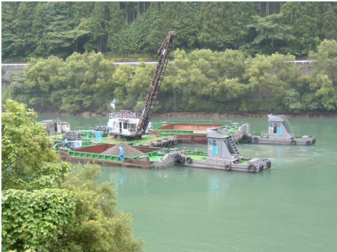
Figure 4-1 Dredging at Sakuma Dam, J-Power
