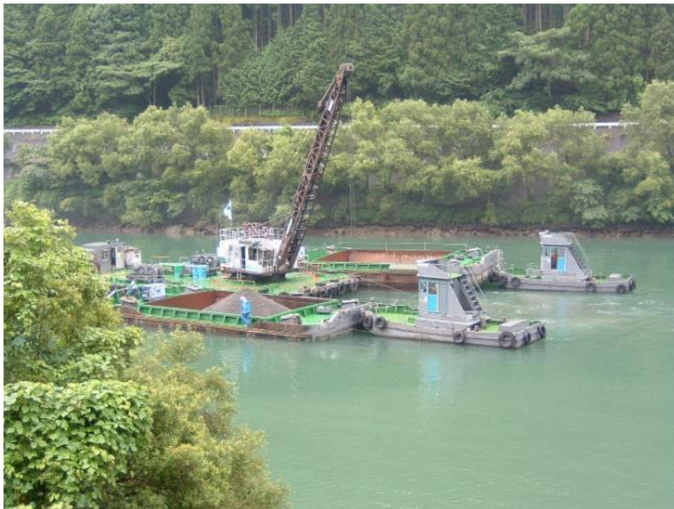
Figure 4-1 Dredging at Sakuma Dam, J-Power
