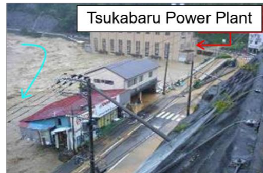
Flooding at Tsukabaru Power Plant
