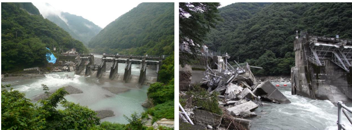
Figure 3-1 Flood Damage Cases at Kyushu EPCO's Kawabegawa No.1 Power Plant (Left: Damage to Intake, Right: Enlarged View of the Right Bank Slope)
