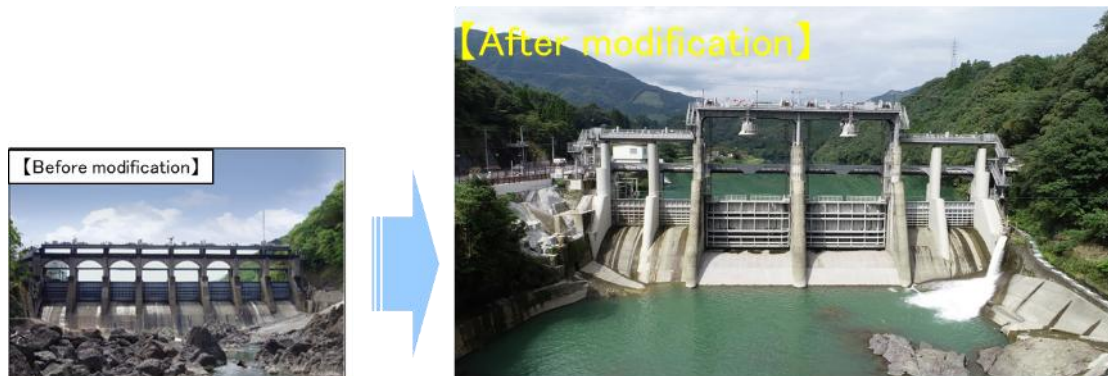
Figure 4-17 State of Saigo Dam Before and After Modifications
