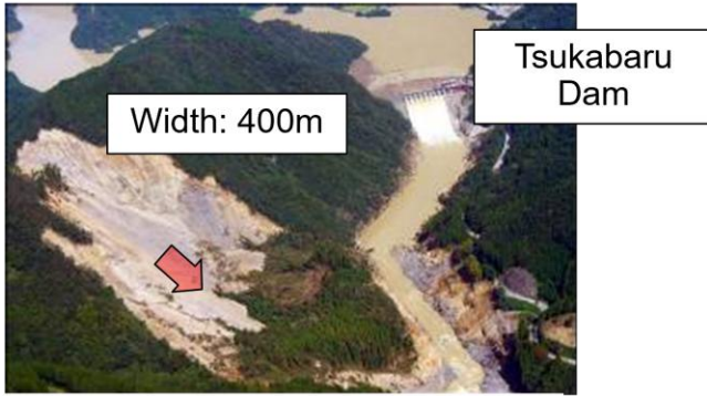
Collapse situation downstream of Tsukabaru Dam
