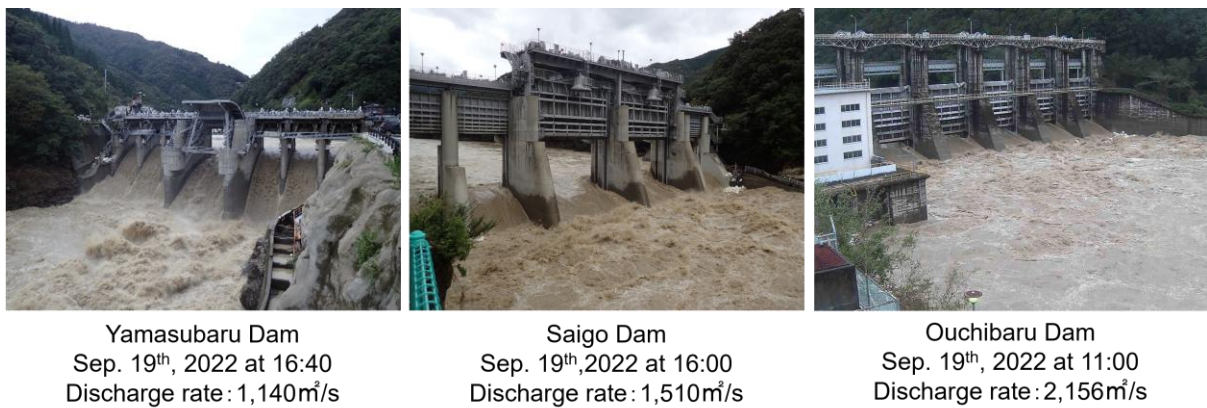
Figure 4-24 Picture of the 3-Dams Coordinated Sediment Flushing Operation
