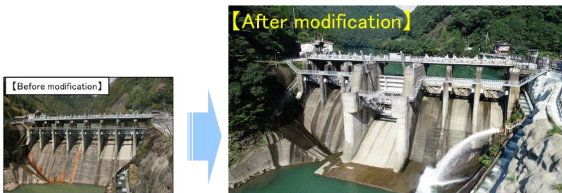
Figure 4-16 State of Yamasubaru Dam Before and After Modifications
